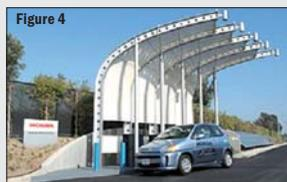
Figure 4: Solar-Powered Water Electrolysis Hydrogen Fueling Station
